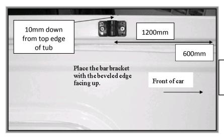
**Figure 2**: Placement of bar bracket
