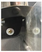
2. Drill 5 evenly spaced holes through the 25mm section of the angle and into the top edge of the tub. The first hole from each end will be about 130mm from the end of the angle. Pop rivet into place with 5 x long rivets.
